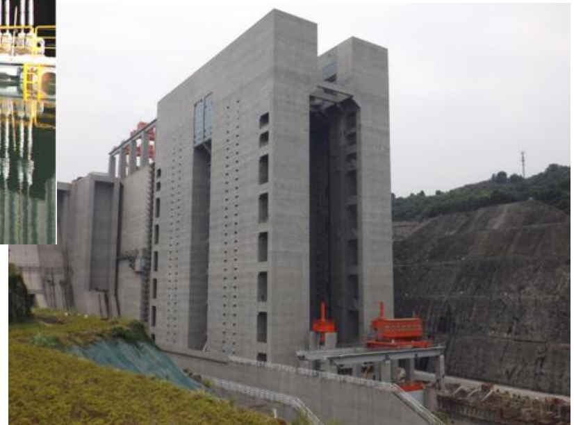
Ship lift after completion
