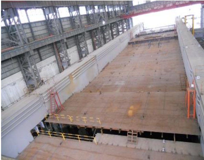
Pre-assembly of ship container (in segments) in the factory
