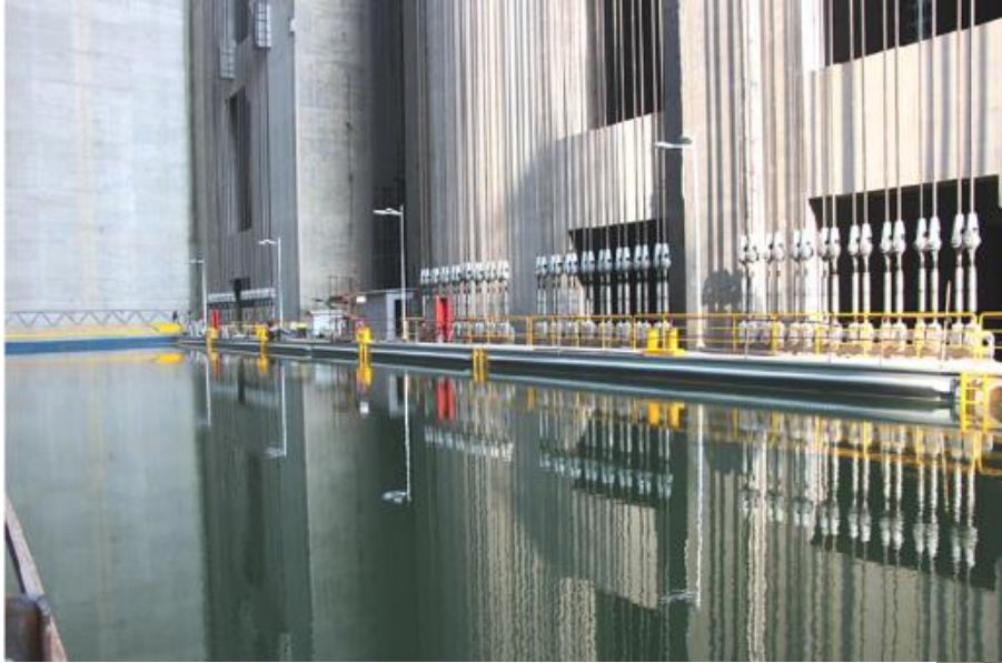
Container of ship lift after completion
